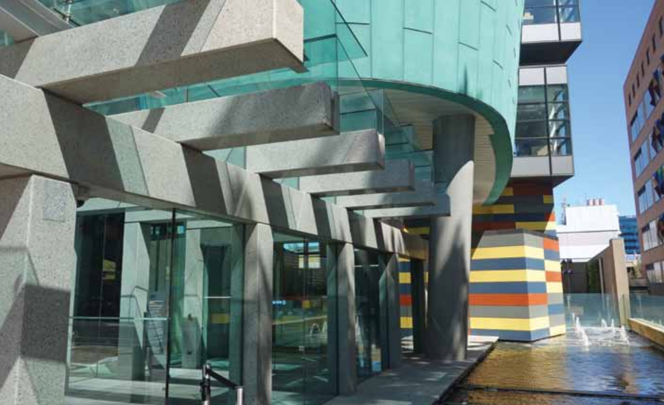
Adelaide: The interesting Commonwealth Law Courts was easier to build as the federal government controlled the land and planning
