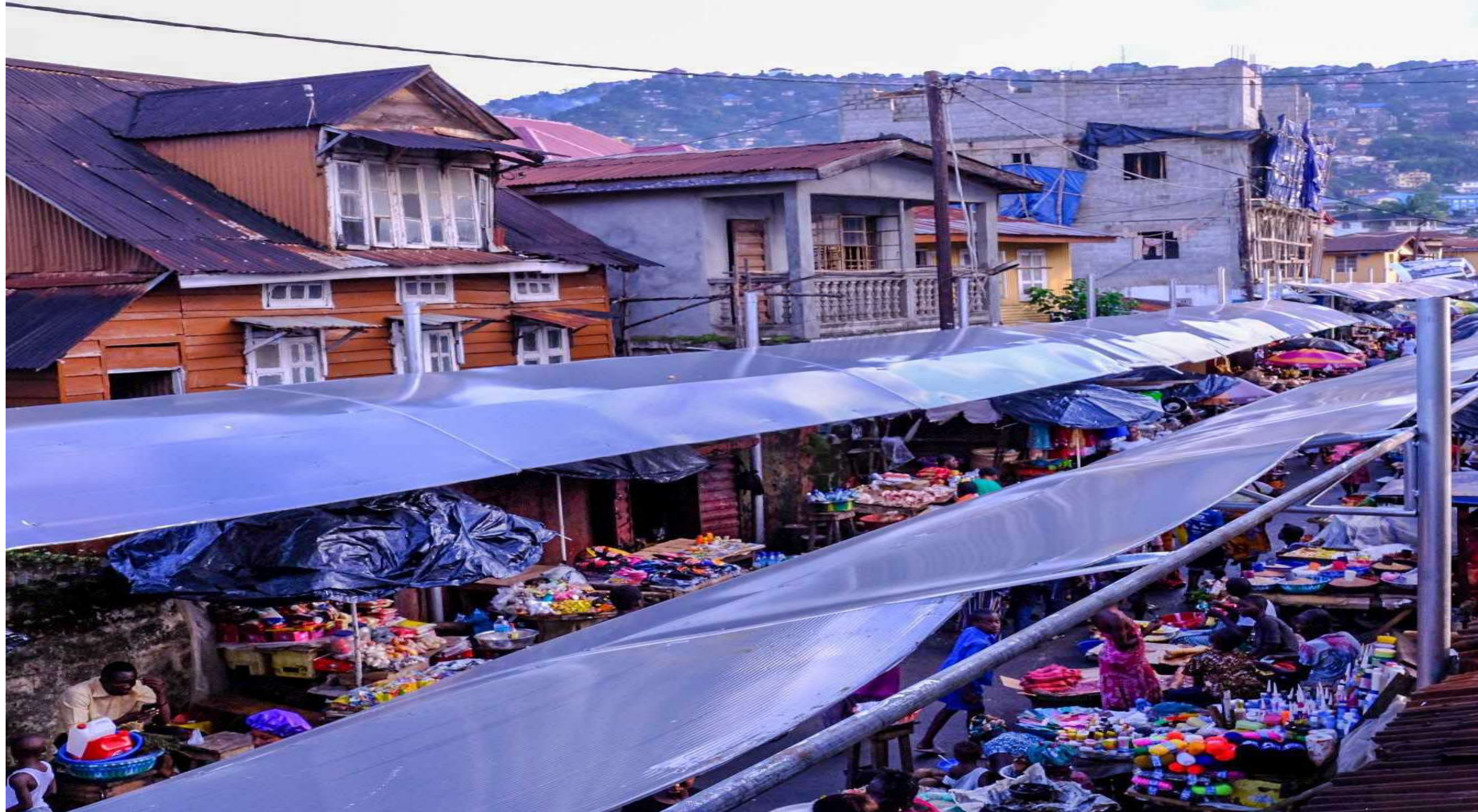
After – Congo Market with its new shade covers installed
